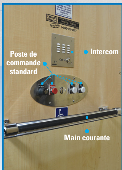
STATION DE COMMANDE
