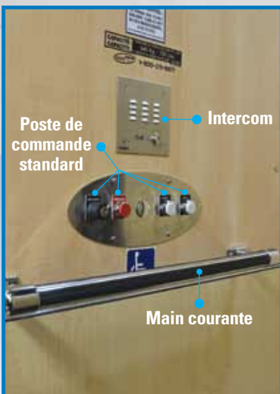
STATION DE COMMANDE
